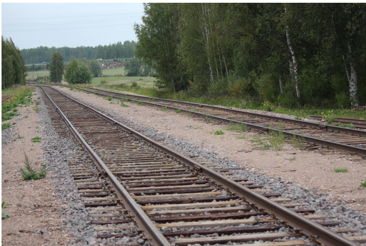
Figure B - 7: Reused wooden sleepers, Lapinjärvi, Finland, August 2021 (source: FTI Finland)
