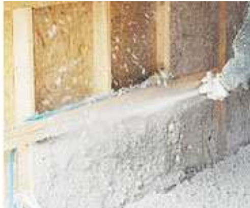
Figure 5: Illustration of cellulose insulation flocking (NrGaia website, 2013)
