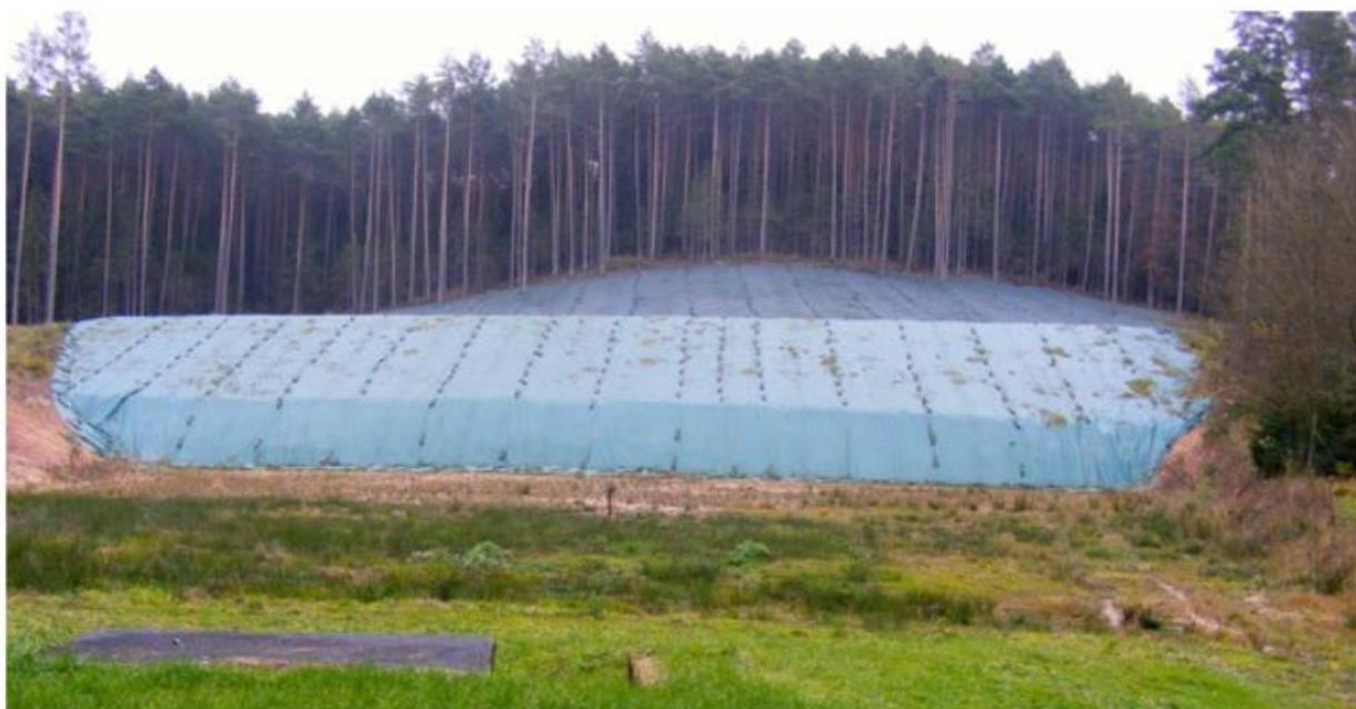
**Figure 1-5: Example of a horizontal barrier (Bavarian LFU, 2014)**
