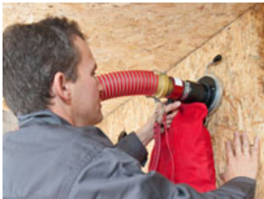
Figure 4: Illustration of injection of cellulose insulation (NrGaïa website, 2013)
