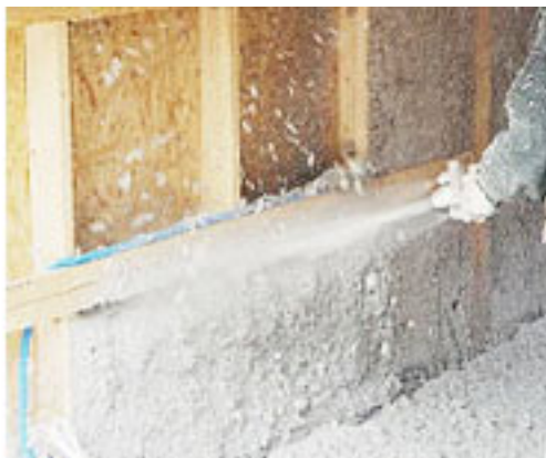
Figure 5: Illustration of cellulose insulation flocking (NrGaia website, 2013)
