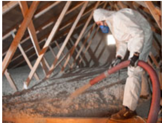
Figure 3: Illustration of spreading in the attic (NrGaïa website, 2013)
