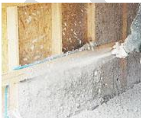
Figure 5: Illustration of cellulose insulation flocking (NrGaia website, 2013)
