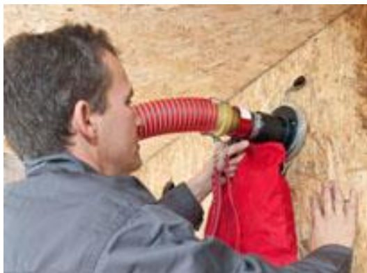
Figure 4: Illustration of injection of cellulose insulation (NrGaia website, 2013)
