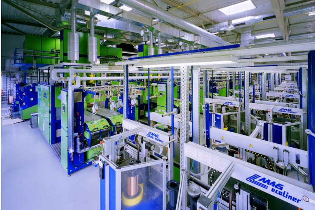
Figure X01.1: Two pictures of enameling machines in a wire coating factory.
